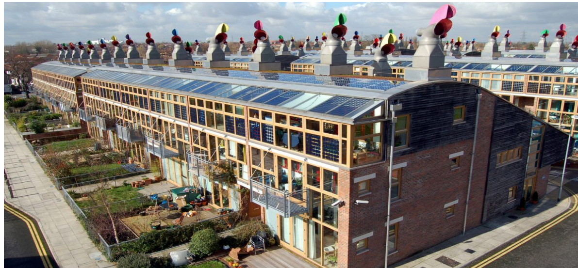
BedZED project sustainable housing, first conceived in 1997
